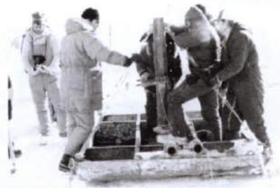
Preparing the discharge sled for lowering to the ocean floor.
